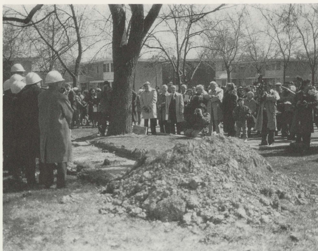
Keiro Nursing Home Groundbreaking
